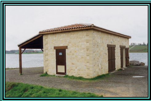
Landscape-friendly compressor technical building
